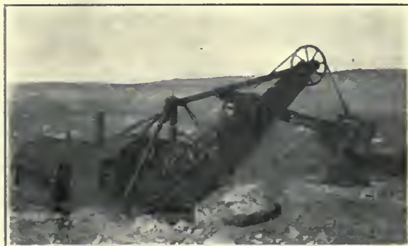
STEAM-SHOVEL STRIPPING A MINNESOTA IRON MINE.
